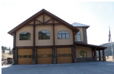
Floyd Hill, Station 6
