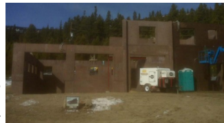
St. Mary's Station 7 Under Construction
